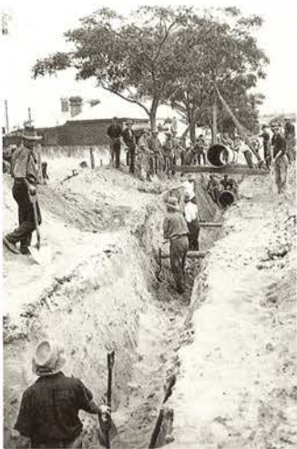
Workers at Humes Ltd, pipe manufacturers, lay pipes in a Perth suburb. The award wage for this kind of work was £3 14s 11d for a 44-hour week. This was 11d higher than the Perth basic wage, the lowest wage legally payable by an employer. Humes Limited papers.
